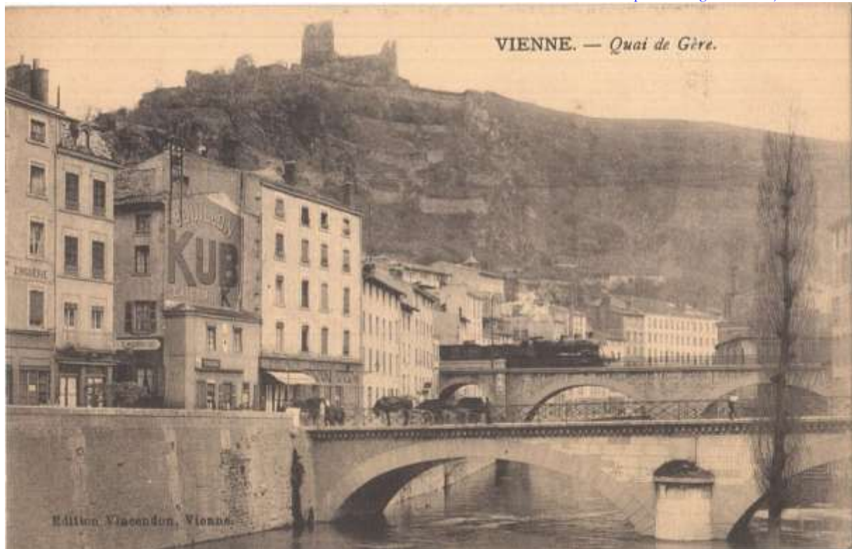
Fig. 6. Partial view of the elevation of the Pont Gère, showing the north abutment and the arch that rests on it (Rue des Quatre – Vents side) and the start of the other arch in the pier, photographed downstream at a time when there was an increase in the rise in the water level (compare with Fig. 2 or Fig. 5), on a postcard from the early twentieth century (Brisaud, 2018, 136).
