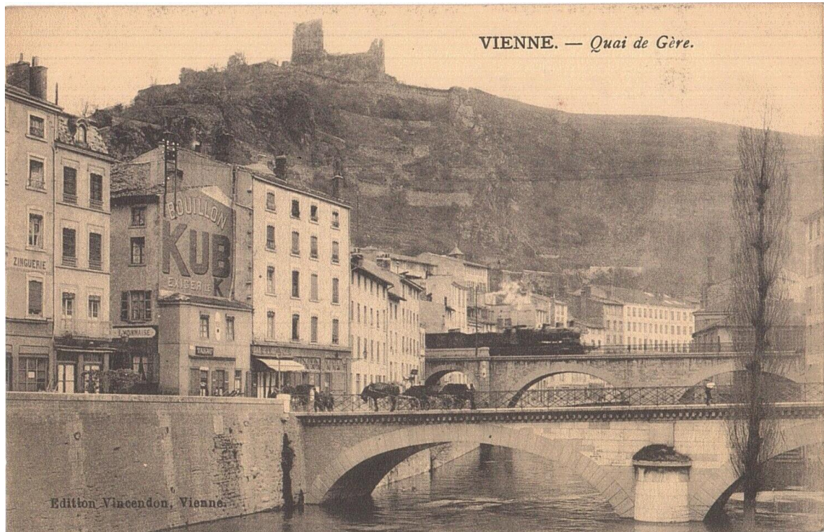
Fig. 6. Partial view of the elevation of the Pont Gère, showing the north abutment and the arch that rests on it (Rue des Quatre – Vents side) and the start of the other arch in the pier, photographed downstream at a time when there was an increase in the rise in the water level (compare with Fig. 2 or Fig. 5), on a postcard from the early twentieth century ( https://i.ebayimg.com/images/g/UbsAAOSw6G9gazSe/s-11600.jpg ).
