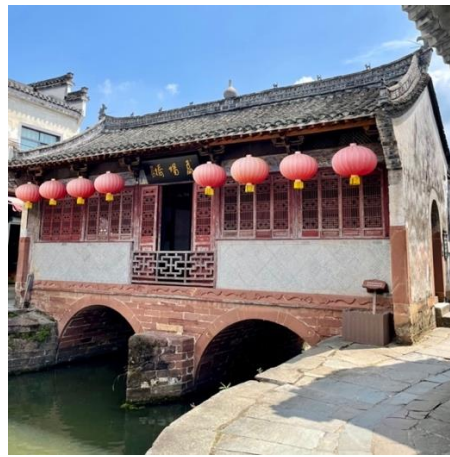
Figure 4. The Architectural Appearance of Gaoyang Bridge
