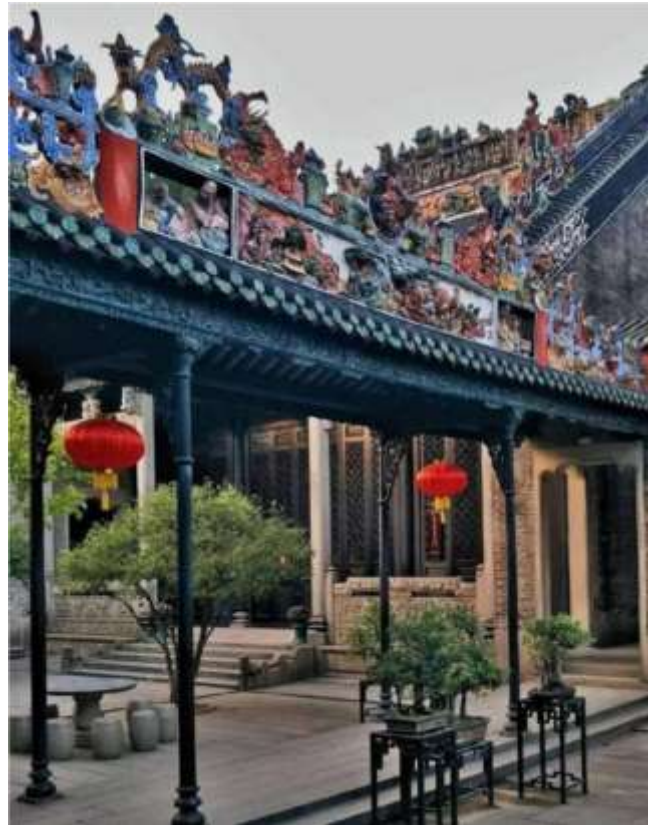
Figure 4: Cast-iron corridor frame, Chens' ancestral temple, Guangzhou
