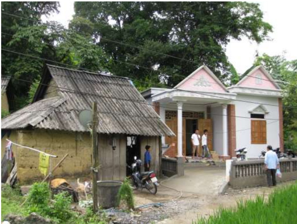
Photo 2. A Semi-Traditional Rammed Earth House Next to A Newly Built Brick House. Quyết Tiến Commun. Quận Bạ District. Hà Giang Province. July 24, 2011. First Author's Photo.
